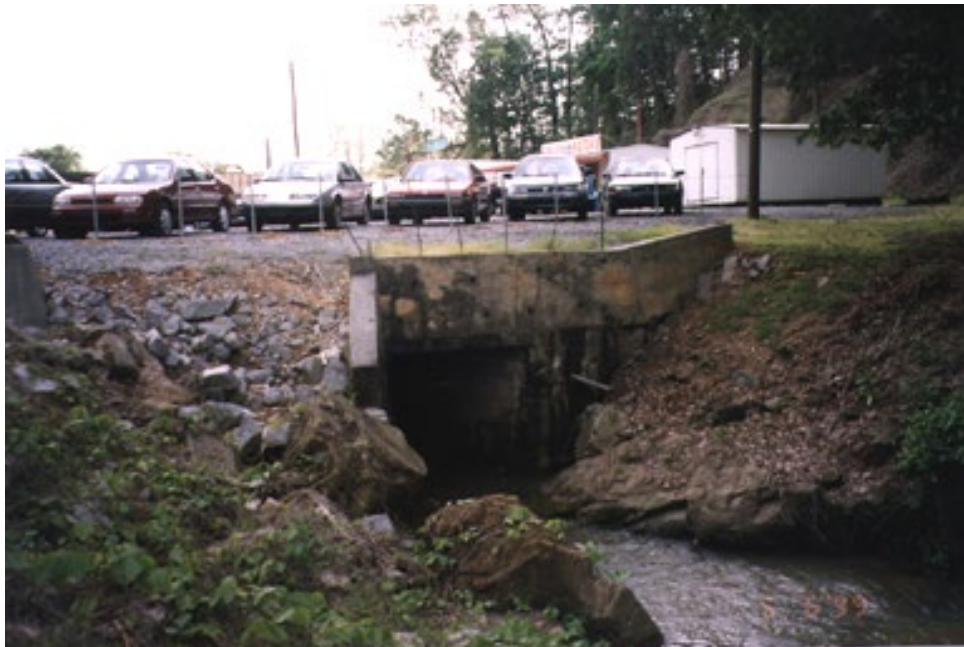
Figure 7-14. Hines Branch at the downstream face of the Amoco Station culvert
