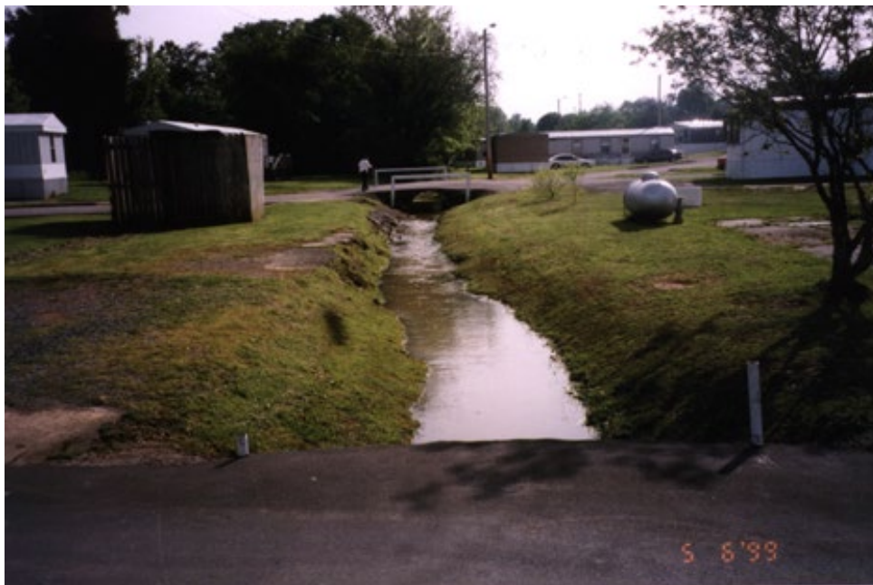
Figure 7-16. Hines Branch upstream of the Trailer Park Driveway #1 culvert (looking upstream)
